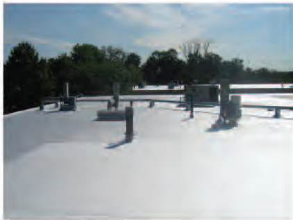
BULLDOG Aluminum Coating application
