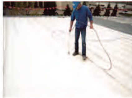
BULLDOG/DUREX Elastomeric Coating application in White.
