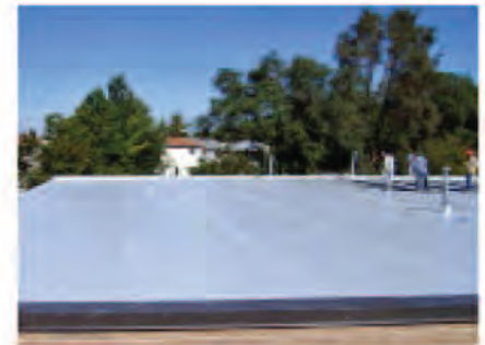
BULLDOG Silicone Coating application
