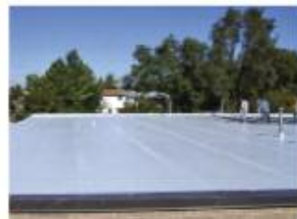
BULLDOG Silicone Coating application
