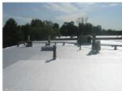
BULLDOG Aluminum Coating application
