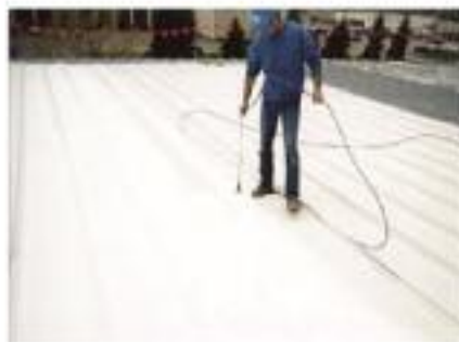
BULLDOG/DUREX Elastomeric Coating application in White.
